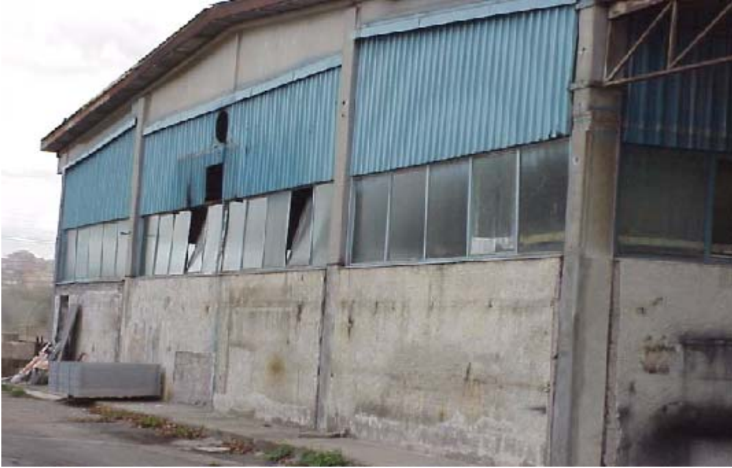
PRE CONSTRUCTION, EXTERIOR BUILDING, LEFT SIDE
