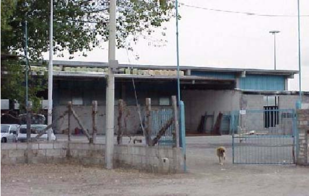
PRE CONSTRUCTION, FRONT ENTRANCE "WITH GUARD" SEPT. 99
