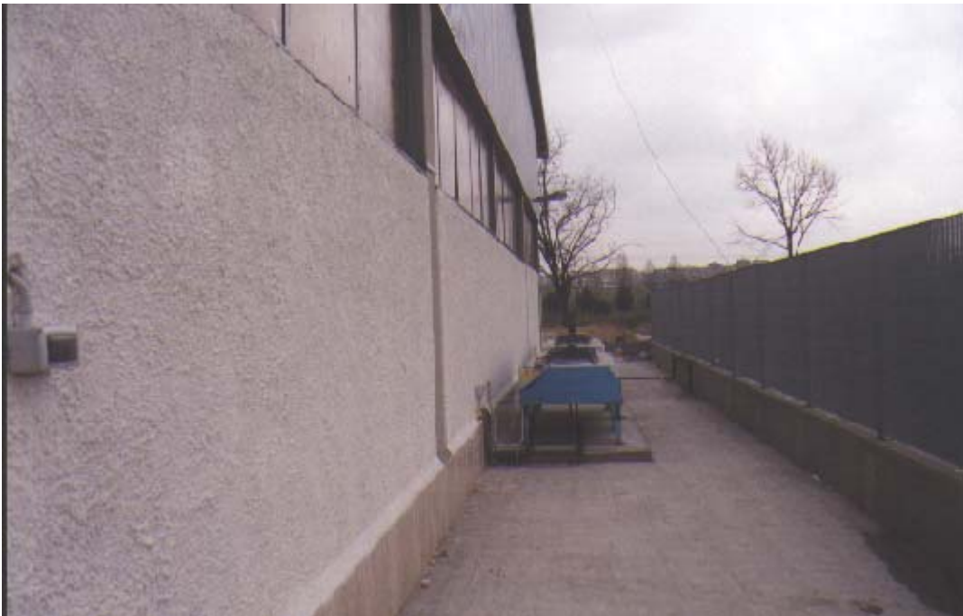
BUILDING REAR AS OF DEC. 99
