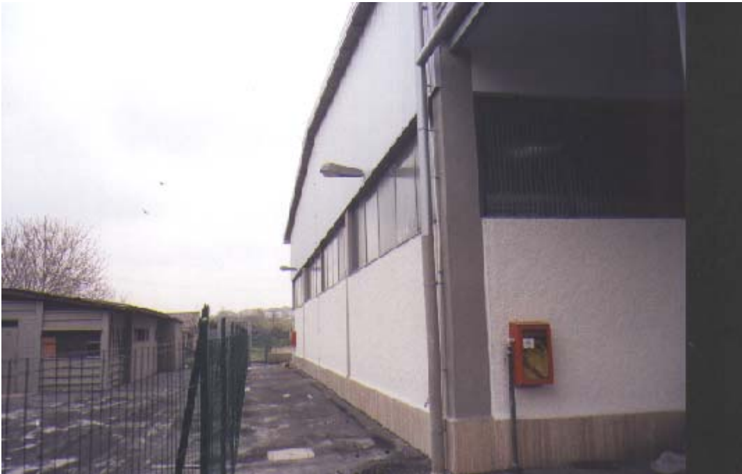
BUILDING EXTERIOR, LEFT SIDE, AS OF DEC. 99
