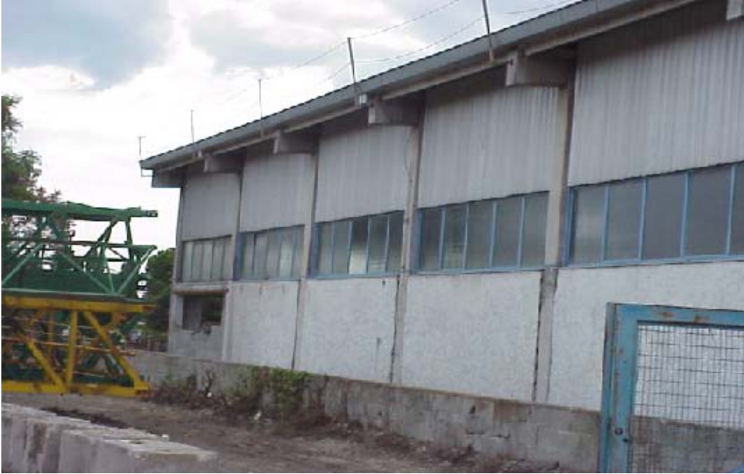
PRE CONSTRUCTION, BUILDING REAR, SEPT. 99
