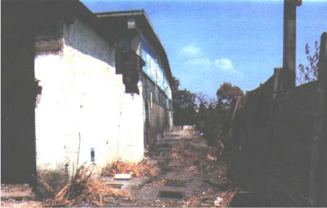
PRE CONSTRUCTION, BUILDING EXTERIOR, RIGHT SIDE, SEPT. 99
